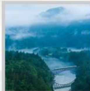
"TADAMI FIRST BRIDGE"
